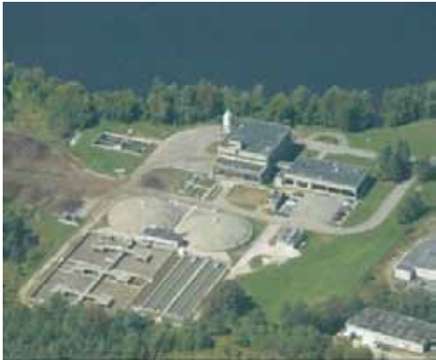
Waste water treatment plant LAWPCA
